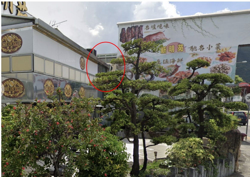
View 2: Existing downpipe location
