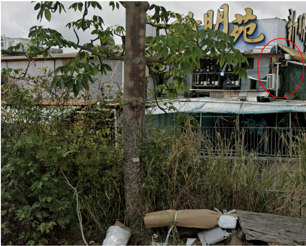
View 3: Existing downpipe location
