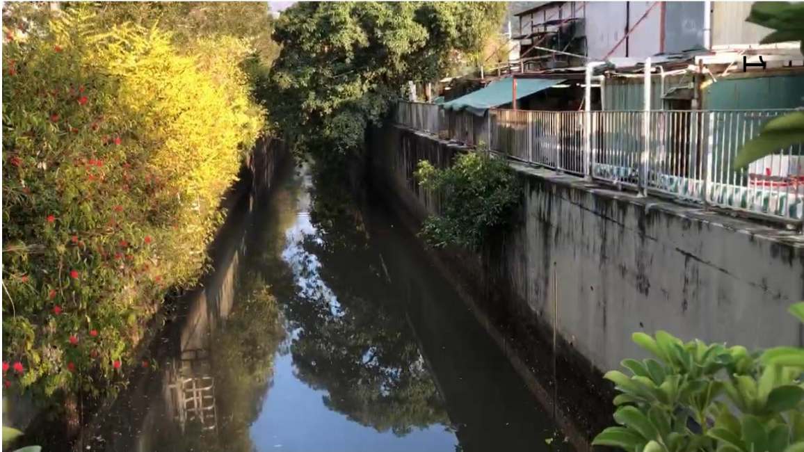
View 1: Existing Nullah condition and downpipe location
